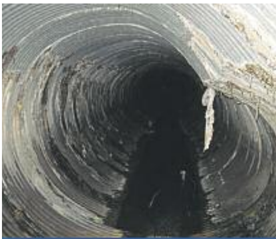
Rheem shopping center culvert for Laguna Creek
